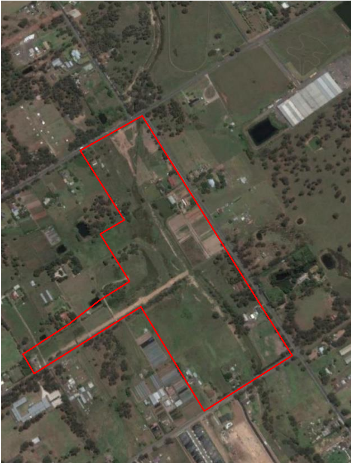
Figure 8: 2015 aerial imagery showing further excavated works for Sydney Water Infrastructure along Regent Street and corner of Clarke and Garfield Road. (Source: NSW Govt. spatial portal) aerial imagery
