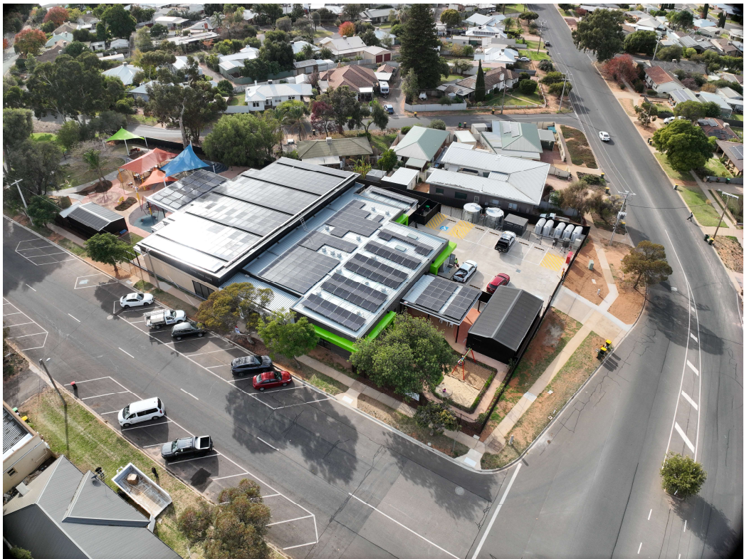
Figure 4: Solar installed at the Red Cliffs Early Years Hub
